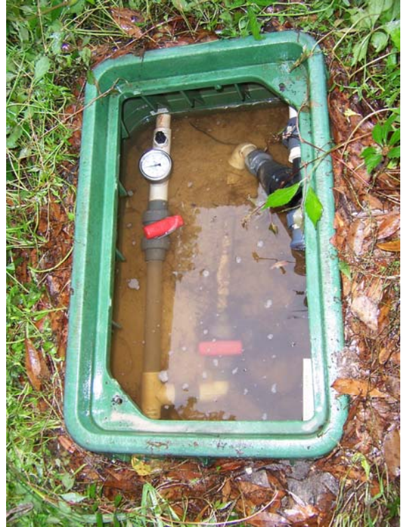
Figure 17. Pictures of site WS-4 taken on April 14, 2009. The broken plumbing evident in this picture was also reported in September 2008. The broken pipe caused the effluent to fill the control box instead of going to the drainfield.
